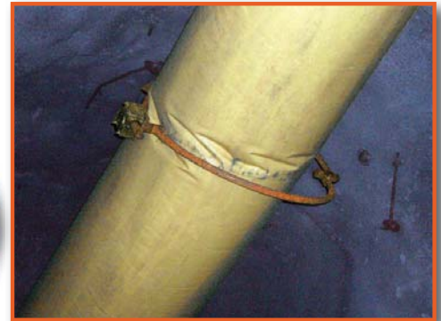
Installed Ventilation Closer
